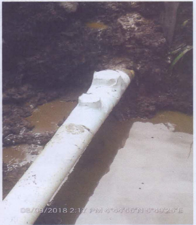
LEAK POINT AFTER REPAIRED
